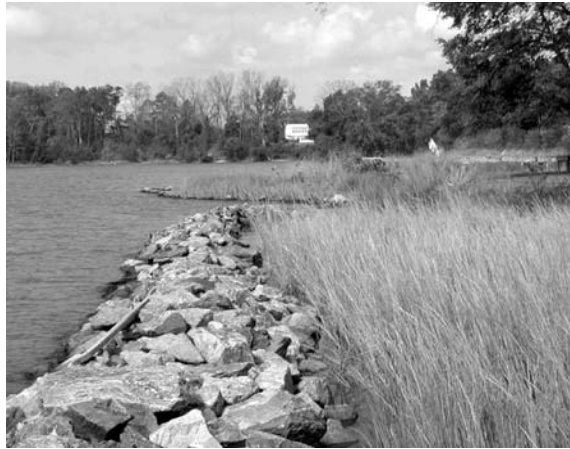
Erosion control using low profile rock riprap with planted marsh.
